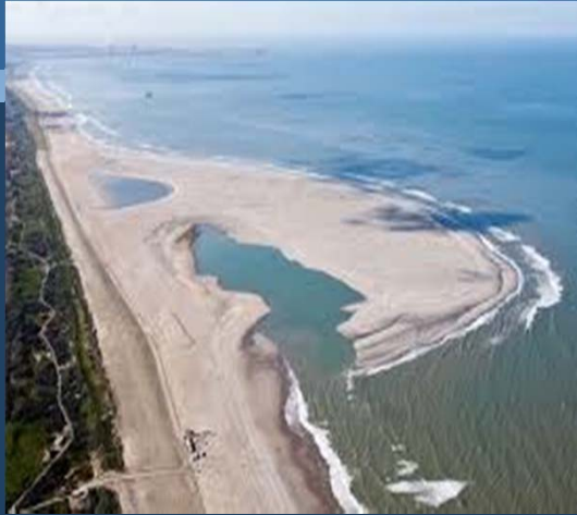
'Sand motor' beach replenishment, Ter Heijde, Netherlands
